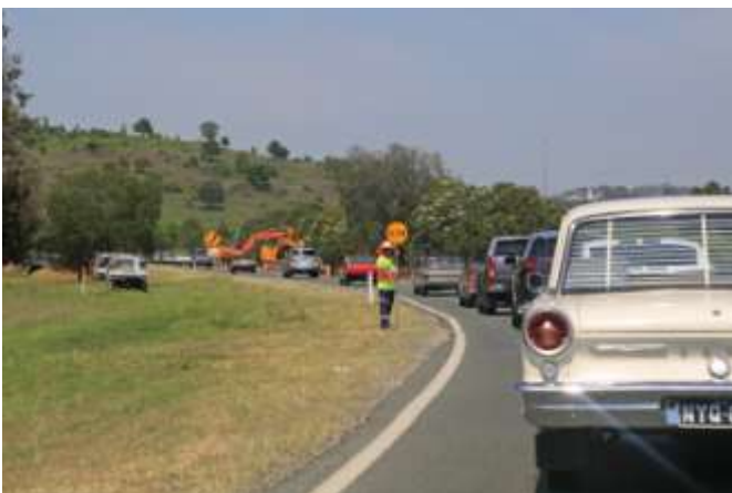
Roadworks and new pipes for Lowood
