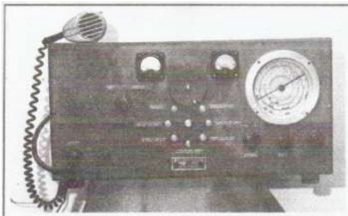
The popular war and post-war Træger vibrator set with power provided by a six-cell high-tension battery. By the mid-war years (c. 1943) the historic pedal generators were replaced by vibrator supplies and Morse code was no longer a necessary provision.
